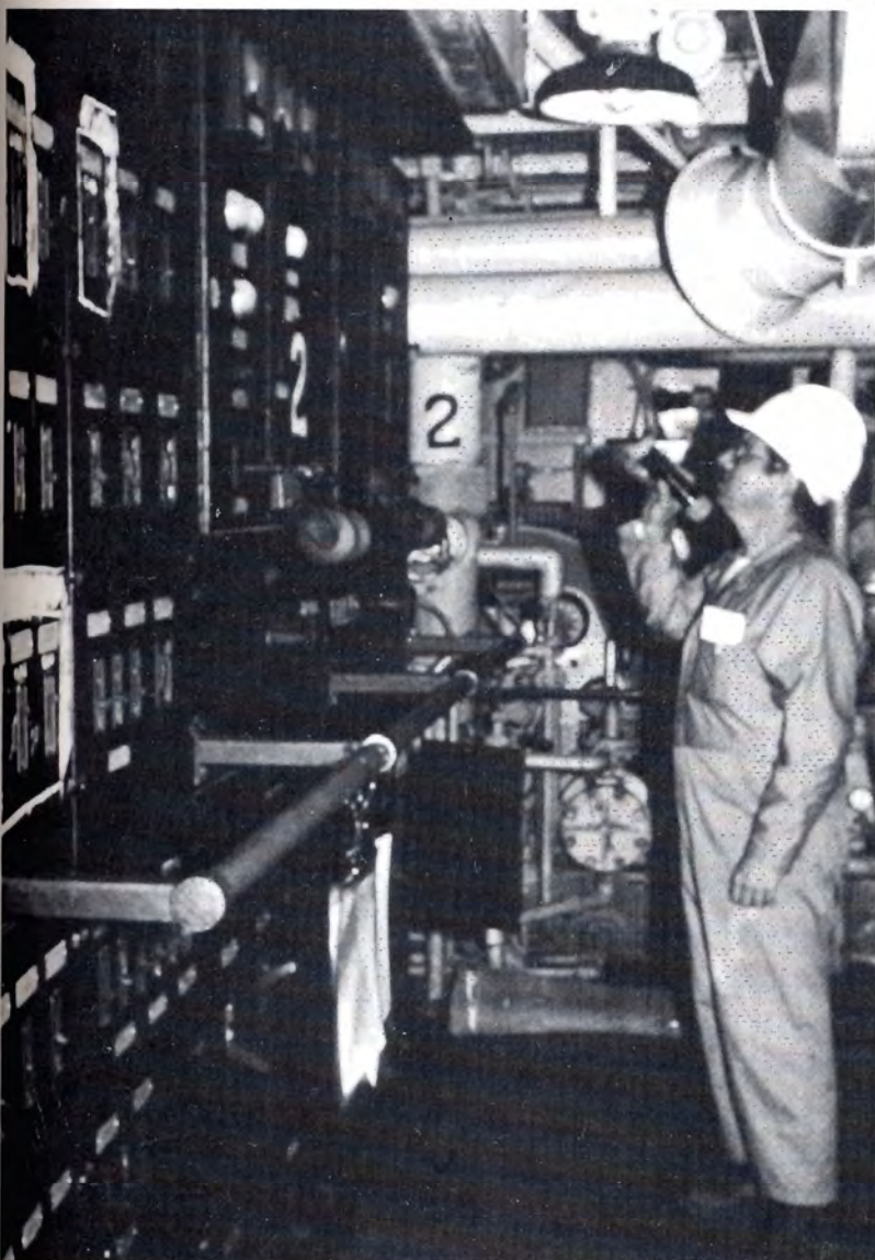
Coast Guard inspector checks electrical generator control board on a commercial vessel.
