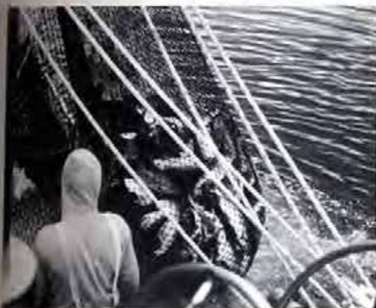
A load of fish is rolled from the seine into the hold. Such operations can dramatically affect vessel stability.
