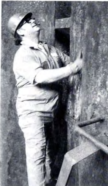
An NCB inspector examines a corrugated bulkhead on a bulk carrier. (Photo courtesy of NCB)
