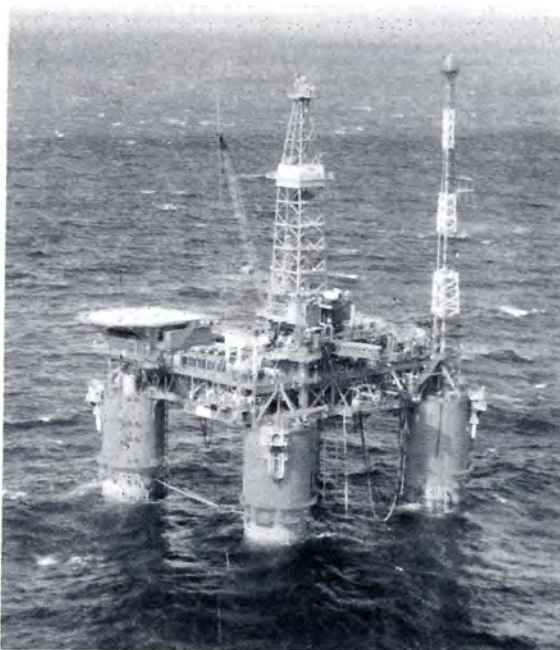
Designs for this tension-leg platform were reviewed by the Marine Safety Center.
