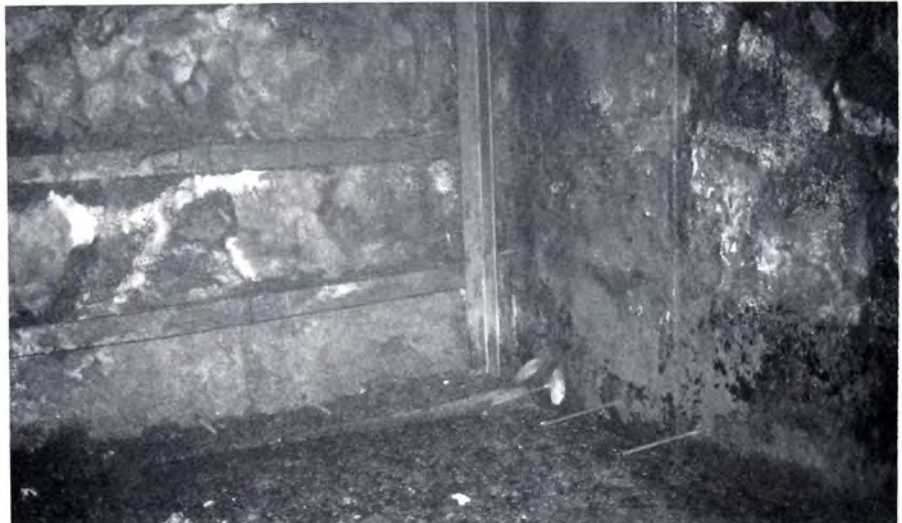
An internal view of the elevator shaft shows the fire damage
