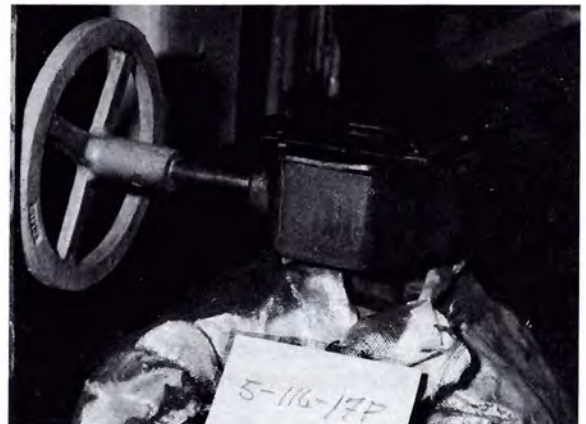
The removal of this cracked gearbox assembly caused the fuel leak that started the fire.
