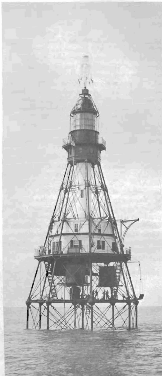
Fowey Rocks in the Florida Keys is a post-Civil War, exposed-site, screw-pile lighthouse.
