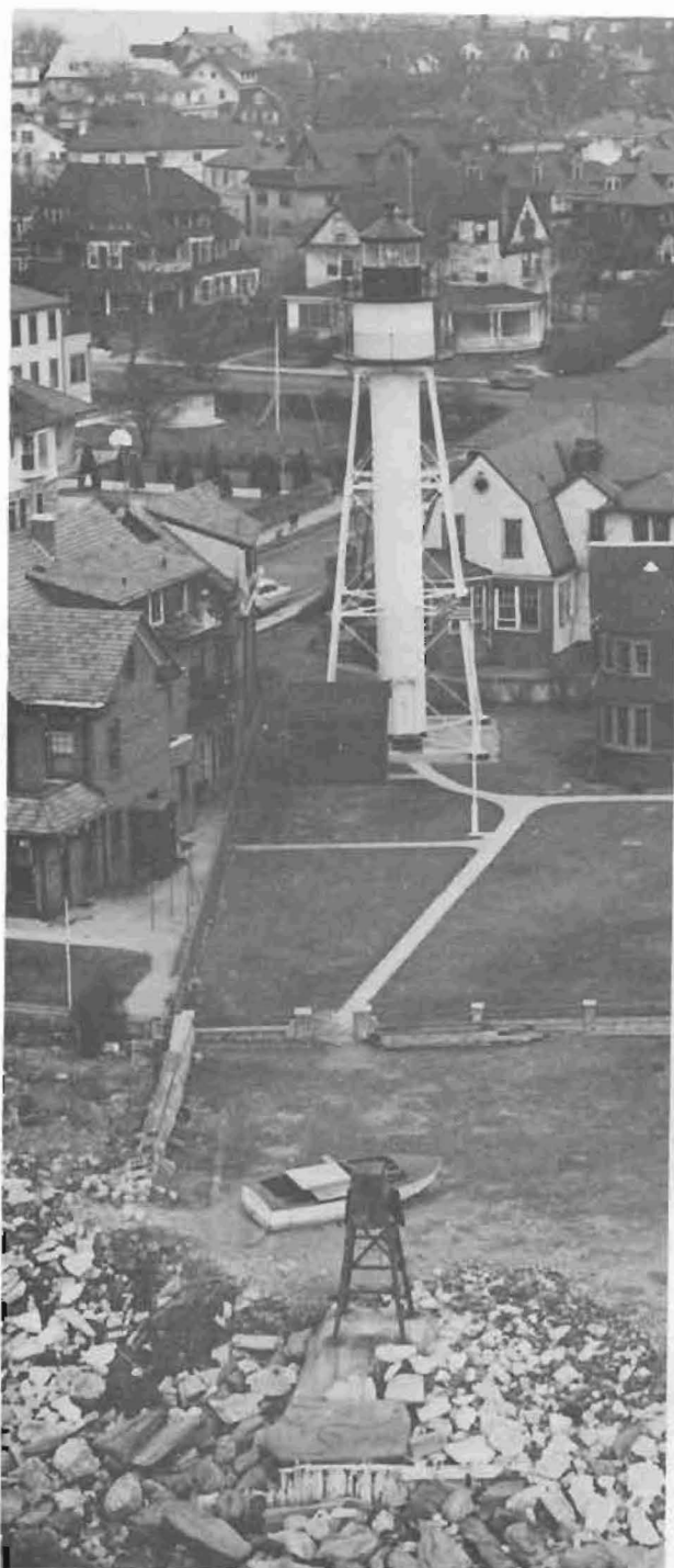
Coney Island, New York, lighthouse is a typical skeleton tower. These towers were built throughout the United States during the late decades of the 19th century and early 20th century.
