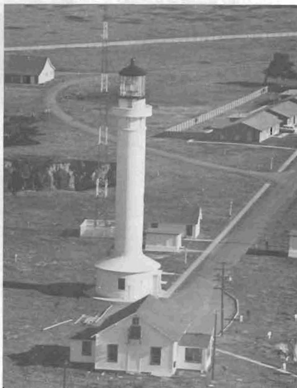
The Point Arena tower in California was the first lighthouse built of reinforced concrete.
