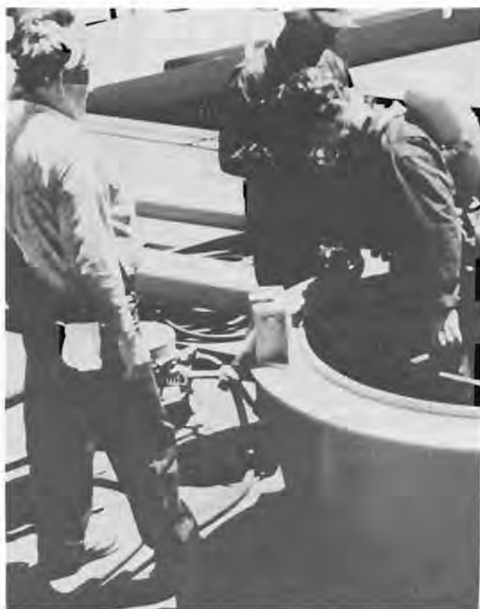
This man is almost properly equipped for tank entry. He is wearing a self-contained breathing apparatus, and he has a support team on deck. He lacks only protective gloves.
