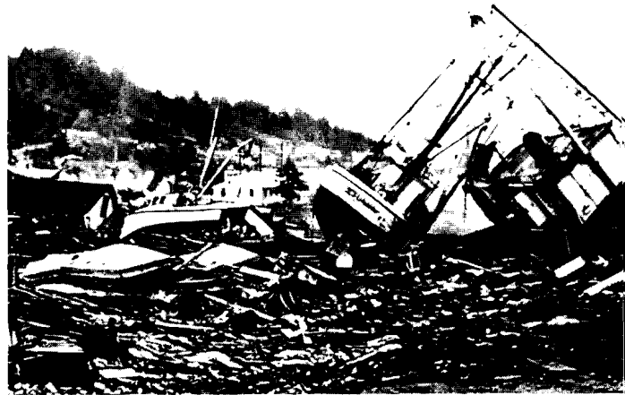
The damage done to the Seward, Alaska, port facilities, like that done to the Texaco truck on the preceding page, was caused by a tsunami generated by an earthquake in Anchorage. Photos courtesy of (left) the U.S. Department of the Interior and (right) NOAA/EDIS
