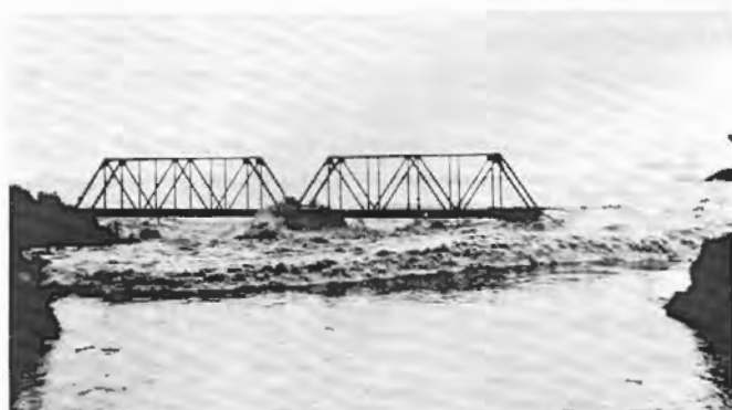
The bore, or advancing wave crest, of a tsunami spawned by an earthquake in the Aleutian Islands passes a damaged railroad bridge over the Wailuka River (Hawaii Island, Hawaii, April 1946). Photo courtesy of the University of California at Berkeley
