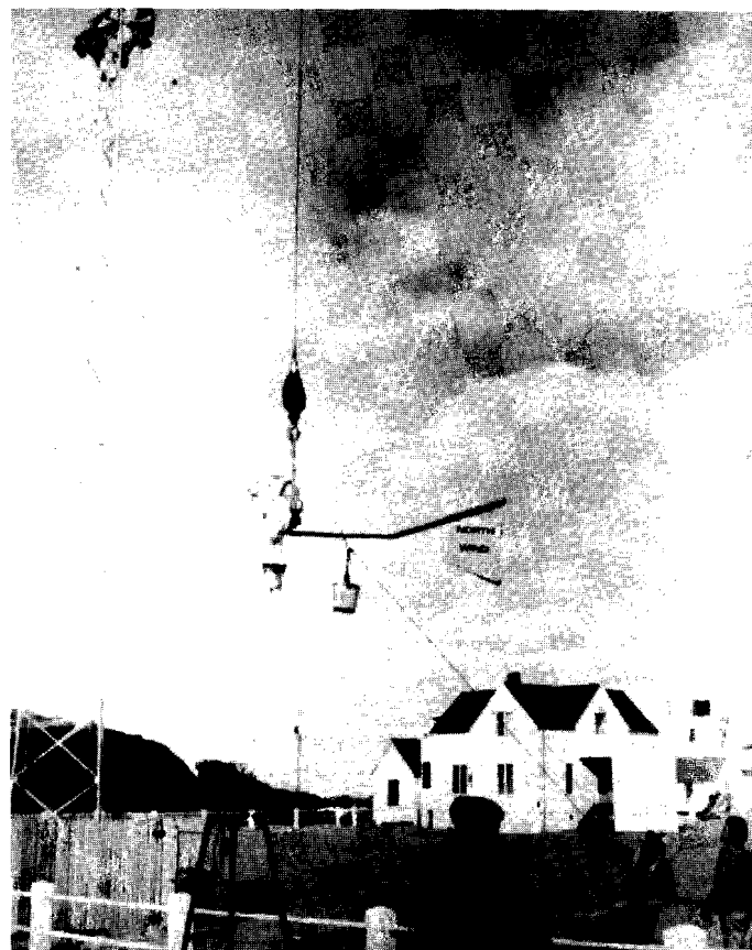
Riggers atop the 60-foot tower prepare to install the wind machine being lifted by crane. The attached bucket was used to lower the tools or other equipment they needed.
