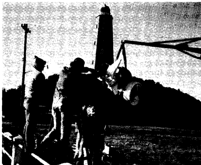
The generator portion of the wind machine is hoisted to a mount prior to the machine's installation atop the 60-foot tower. In the background is the original Cape Henry lighthouse, now a historical monument.
