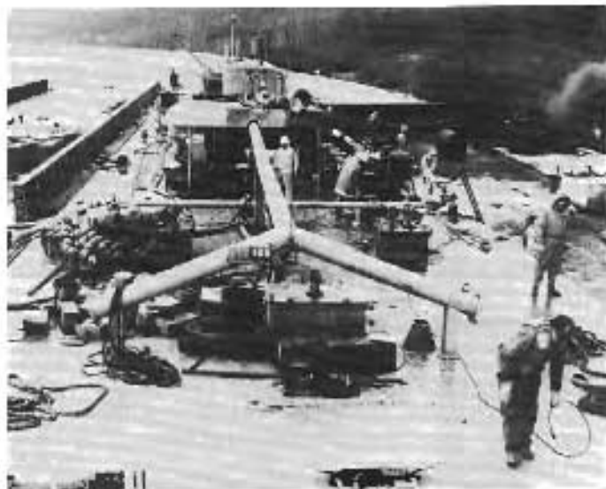
get their equipment in place for the offloading of a barge.
