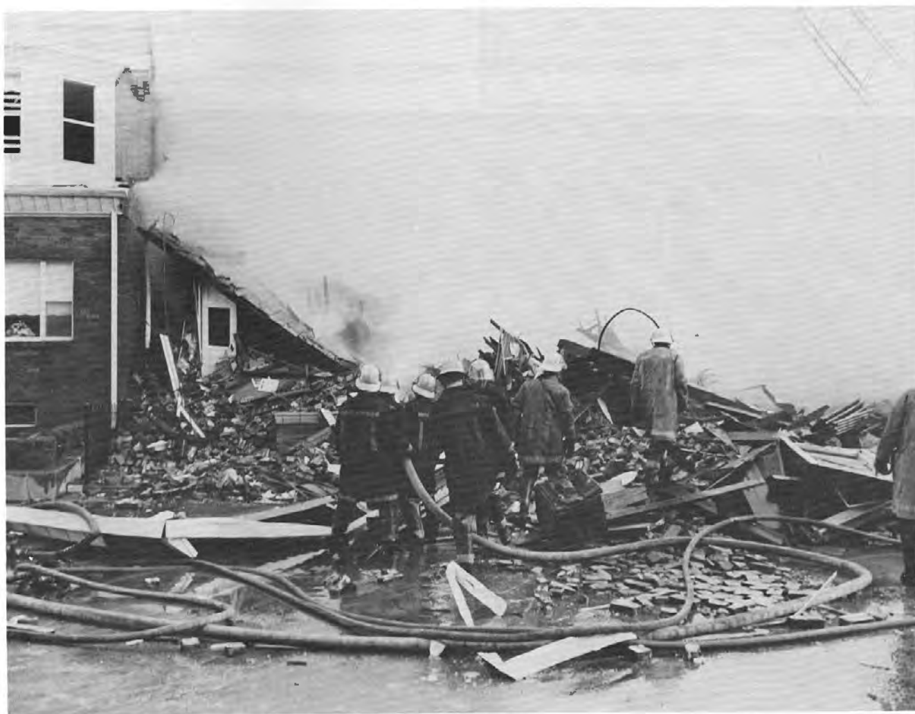
Aftermath of a natural gas burning - an explosion (photo courtesy of National Transportation Safety Board).
