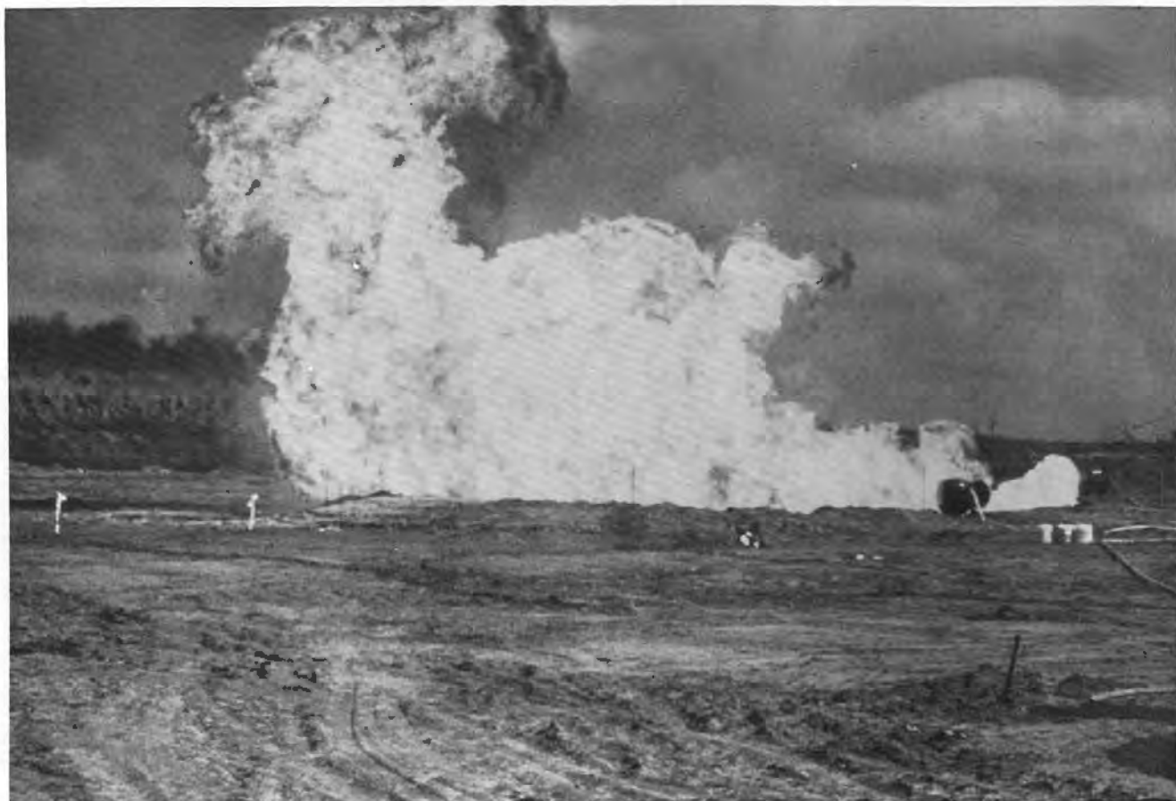
Liquefied natural gas (LNG) vapors burning - a deflagration.
