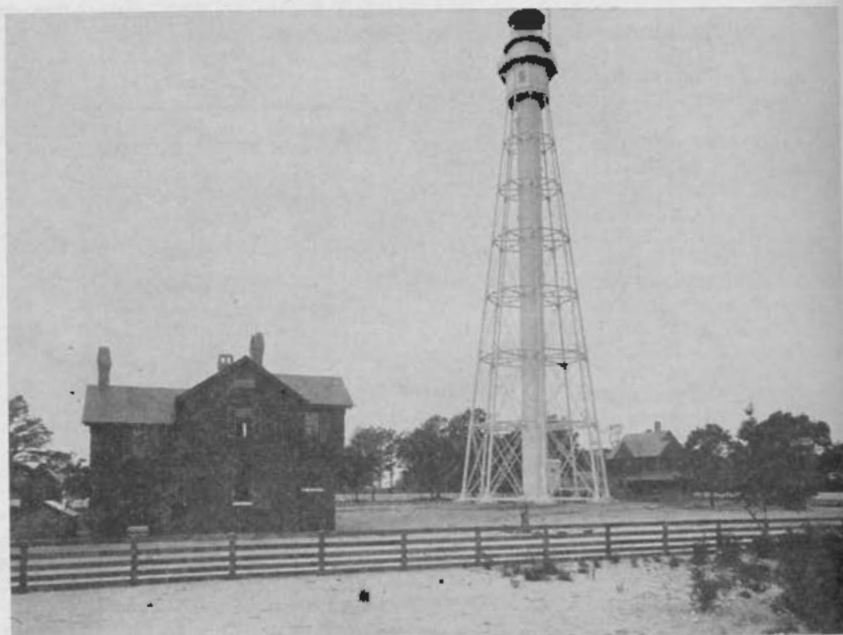
ABOVE PICTURE, taken in July of 1895, shows the then just completed Cape Charles Light Station on Smith Island, Va. The huge first order, 16-panel lens, together with its operating mechanism, has been dismantled and donated to the Mariner's Museum in Norfolk, Va., where it will be installed as an exhibit. The lens cost approximately $20,000 at 1895 prices. The tower is an octagonal, pyramidal skeleton steel structure, with vertical members, struts, and diagonal tie rods. The center is an iron cylinder with an interior spiral staircase. The tower is 191 feet high. The lens will be replaced by a searchlight beacon, atop the tower, which will be operated automatically, and the station will now be unmanned.
