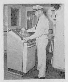
SHIP'S OFFICER plots relative course on the face of a radar indicator unit in the wheelhouse.
