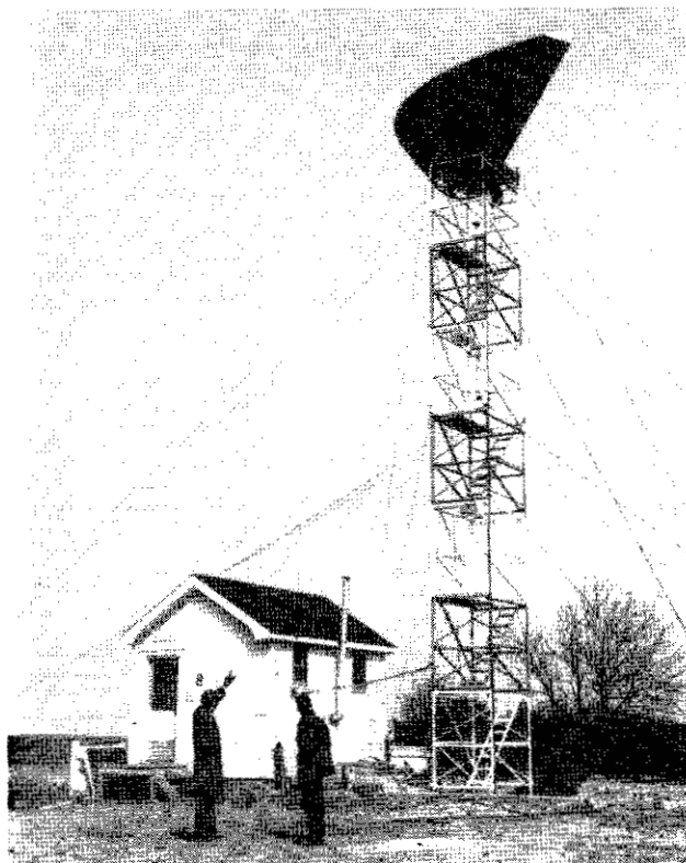
SCANNING LOWER NEW YORK BAY from the tip of Sandy Hook, N.J., this 25-foot-long, boomerang-shaped antenna of a special Raytheon radar sends out electronic signals that come back as high definition echoes. The radar surveys busy area from The Narrows to Ambrose Lightship.
