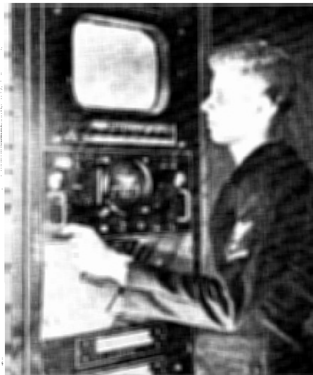
MOVING VESSELS APPEAR with wake-like trails on the converted radar picture so that each ship's course and speed can be estimated at a glance. This is made possible by Raytheon storage tube that remembers positions of targets as they were previously reported by radar. A Coastguardsman checks the transmitted TV picture as it goes "on the air" over Channel 47 from the Coast Guard's experimental RATAN station at Sandy Hook, N.J.
