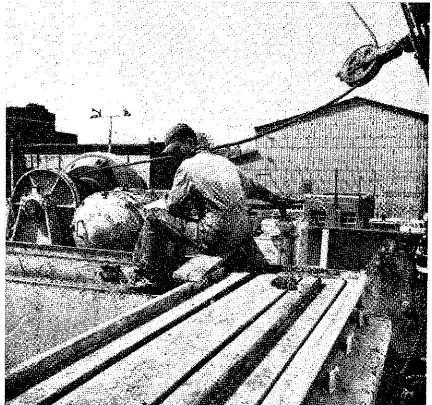
SECTION 9.53(a)(6) of the Safety & Health Regulations for Longshoring prohibits the use of temporary seats for winch drivers which create a hazard to the winchmen. This photo shows a broken, teetering board being used as a seat by a winchman who must straddle the hatch coaming to enjoy this "comfort."
