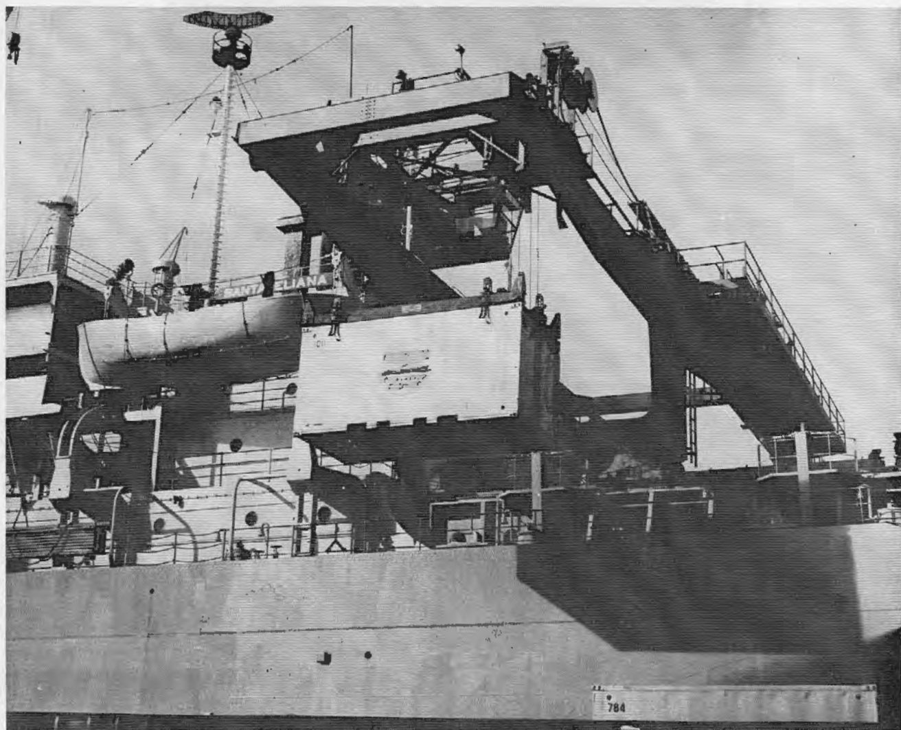
GANTRY CRANES lifting containers aboard the Santa Eliana —first all-container ship in U.S. overseas trade and scheduled to operate in the new Grace Line—Seatrainer Service between New York and Venezuela. (Photo courtesy Grace Lines.)
