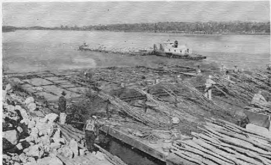
RIVER CREWS WEAVE willow mattresses for protection against erosive action. When completed this mattress will be lowered against the river bank and kept in place with rock fill. Note all workmen except the on-looker in the left foreground are wearing life preservers. Photo Courtesy Corps of Engineers.
