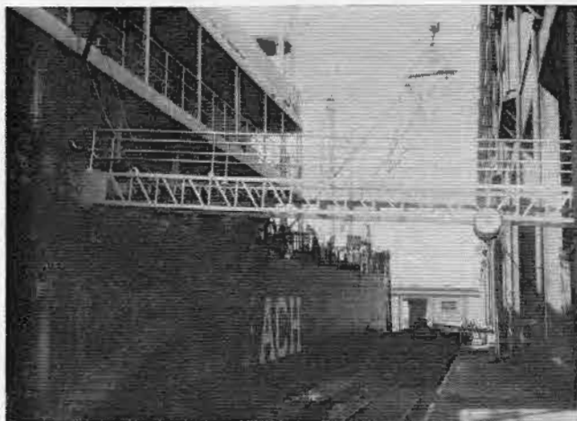
THE OLD AND THE NEW: Looking forward on this C-3 type vessel can be seen Luckenbach's method of solving the problem of sunken tracks and railroad cars between the ship and dock. The ship's gangway is landed on the string piece for illustrative purposes.
