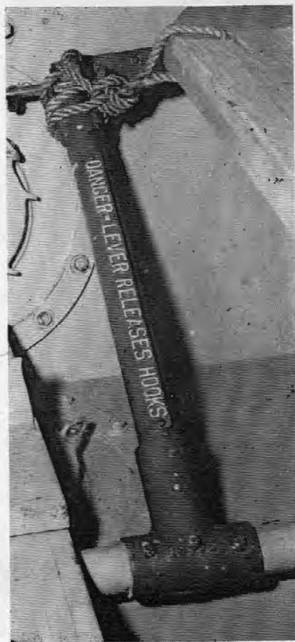
SEEN ABOVE is a Rottmer type release gear handle properly secured in place by toggle pin and several turns of small line to prevent the inadvertent operation of the installation.
