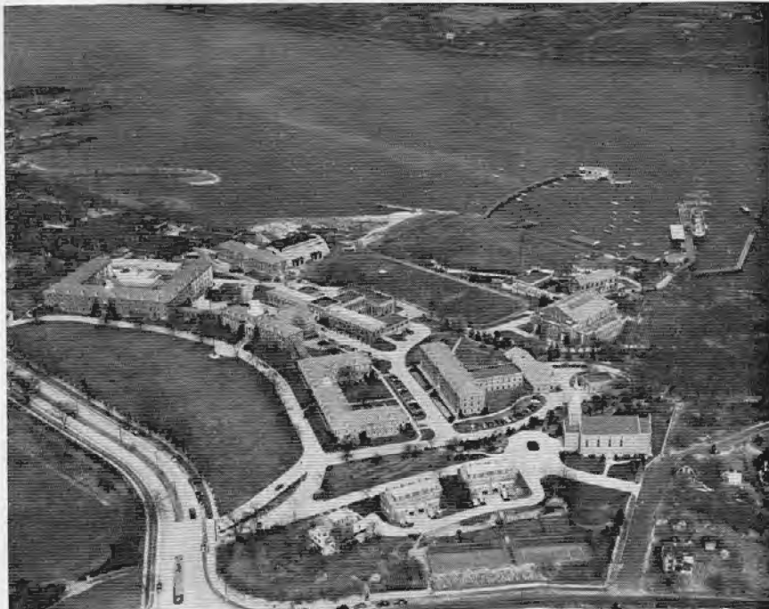
AN AERIAL view of the U. S. Coast Guard Academy, New London, Conn., where future officers of the nation's oldest seagoing force are trained.
