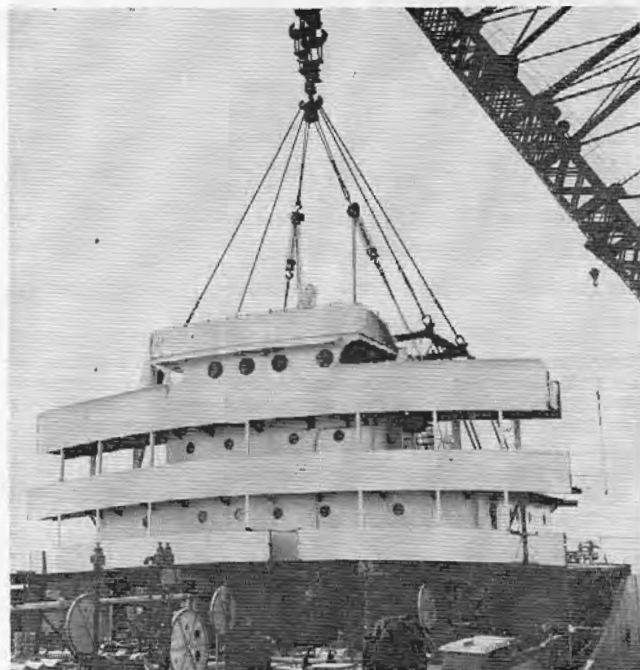
THE DECKHOUSE is placed on new cargo section.
