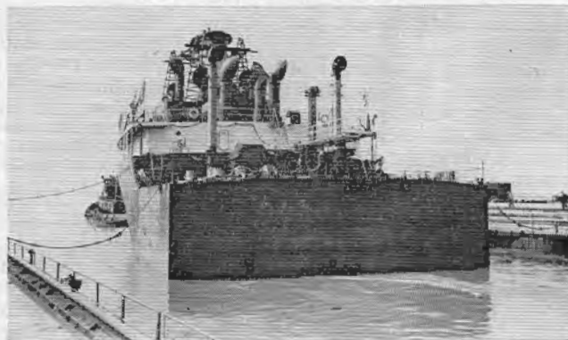
STERN SECTION towed from dock.
