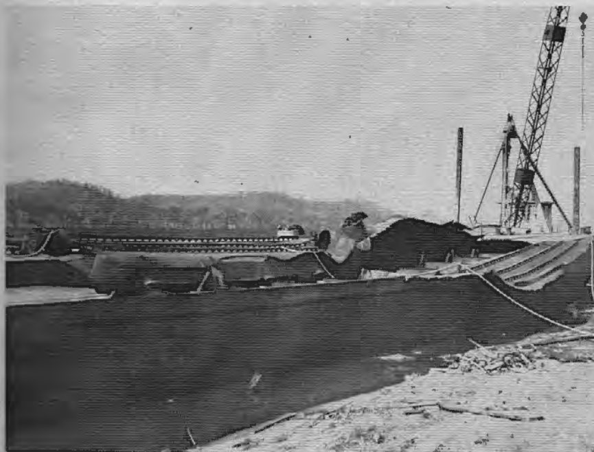
Figure 2. Main deck of tank barge showing effects of vapor explosion.
