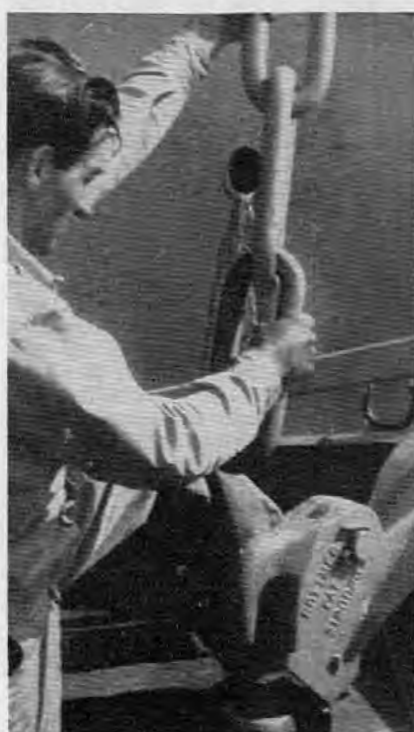
Figure 2. Hooking on lifeboat without using canvas sleeve to cover links.
