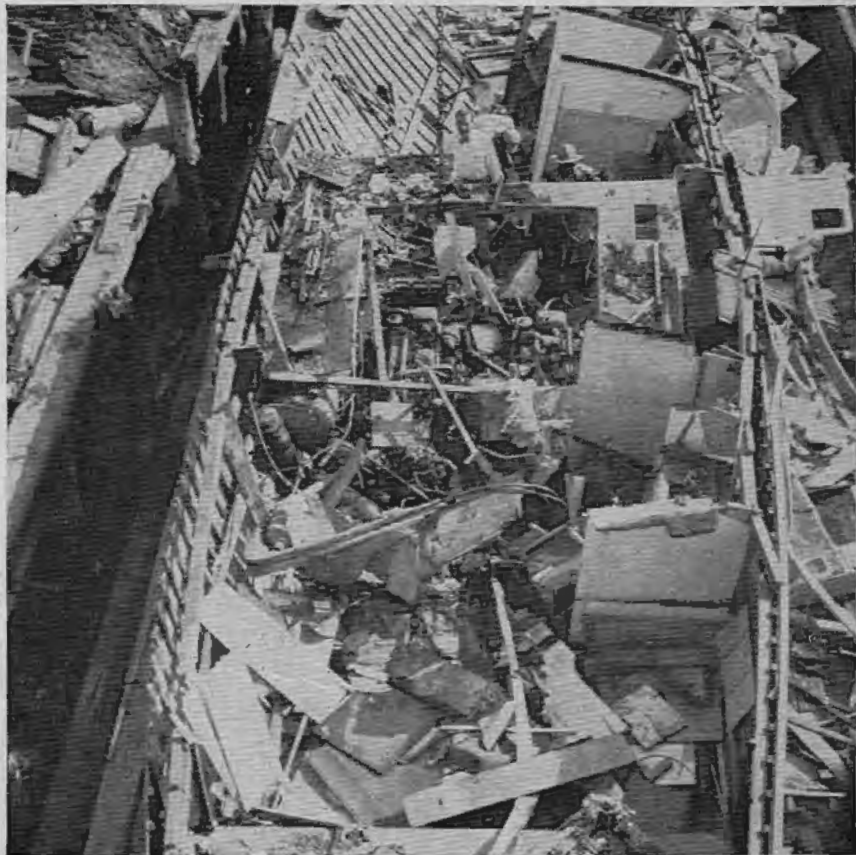
Figure 2. Drip pans were ineffective and permitted gasoline to drip into the bilges.
