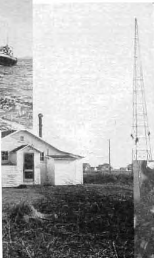
The shack at Marshfield, Mass., where WOU broadcasts to vessels at sea from three 165-foot towers are in the process of being repainted.
