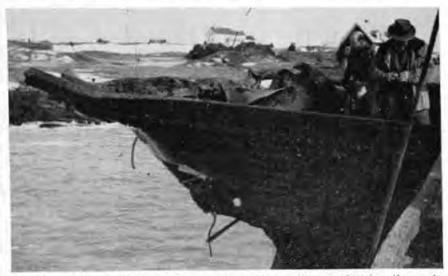
Coaming of No. 4 hatch, starboard side looking outboard, showing the main deck curled up under the force of damage.
