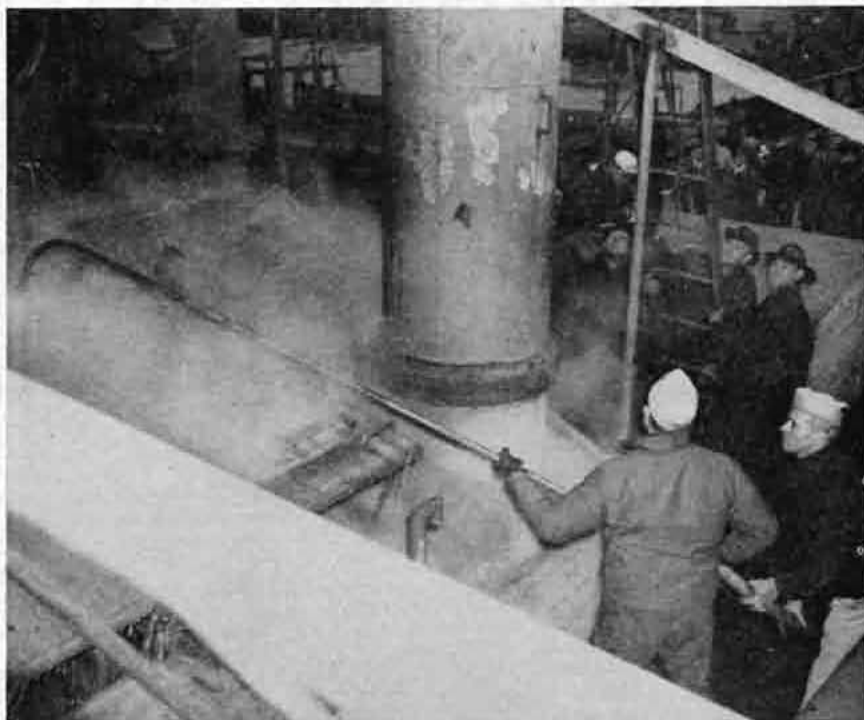
An applicator is used to cool a skylight before covering it with canvas to choke off the air supply as the first step in combatting an oil fire in the engine room. This was one of the new methods studied at the Coast Guard Training Station, Fort McHenry, Md., where a Liberty ship was used for tests under actual conditions.
