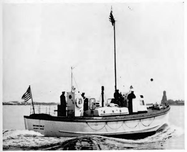
struction is of the strongest. The main engine is a 150 horsepower Diesel with reduction gear. A 3-kilowatt Diesel generating set furnishes electricity. The boat is equipped with radio and searchlights, and all compartments are heated for winter operations. Approximately
