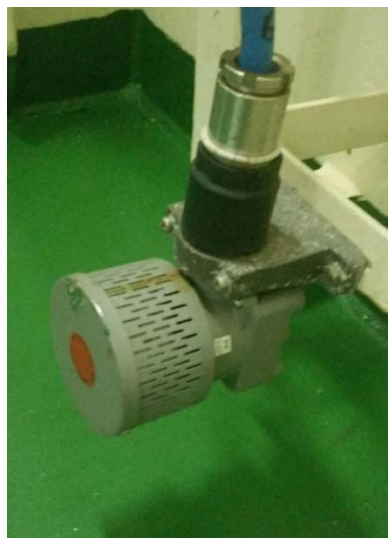
Figure 5-7 Electronic sensor sample point
