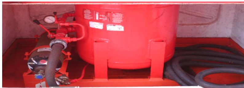
Figure 14-3 Dry chemical powder fire extinguishing system
