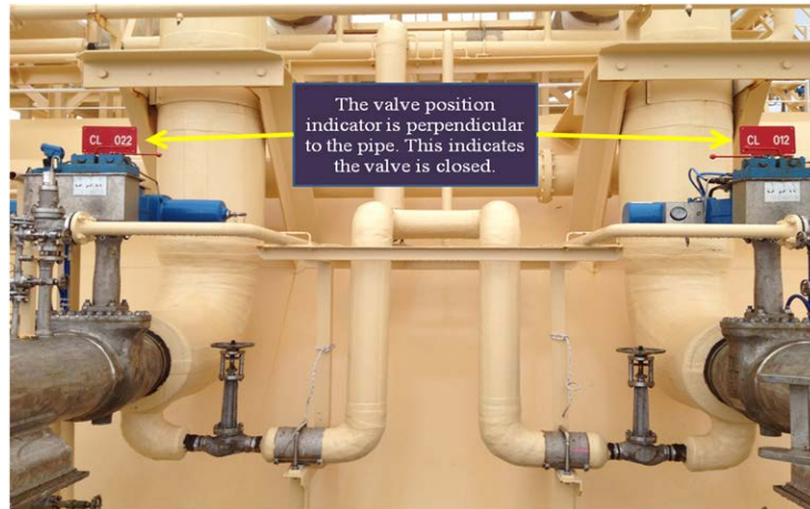
Figure 8-5 Valves position perpendicular to the pipe
