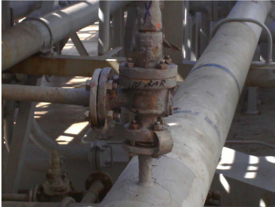
Figure 8-16 Electrically bonded relief valve
