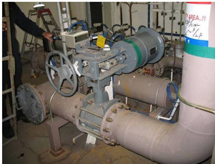
Figure 13-5 Example of second fail-closed shutoff valve installed in series with the MGV in the boiler hood or gas room
