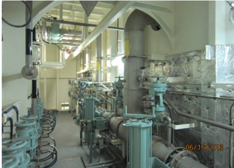
Figure 13-9 Gas utilization room on LNG gas carrier
