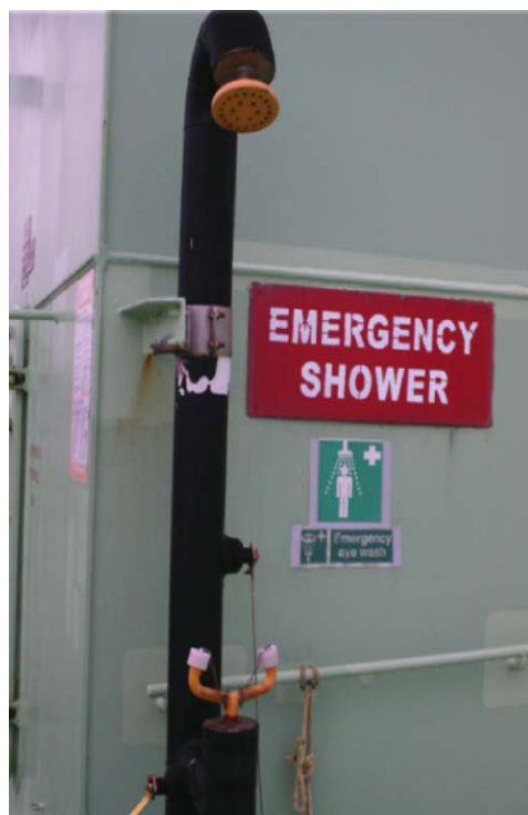
Figure 6-1 Suitably marked decontamination shower and eye wash station
