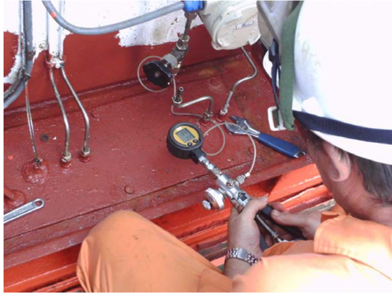
Figure 5-17 Testing of the high/low pressure alarm using a hand pump
