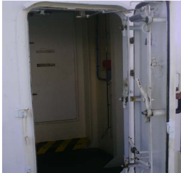
Figure 7-1 Air lock (note the two steel doors)
