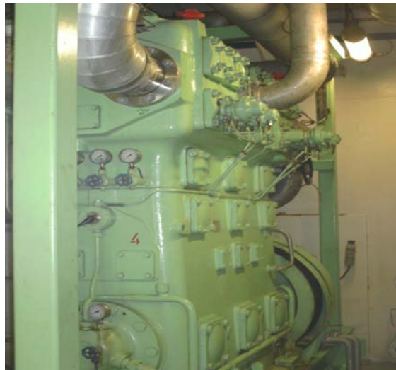
Figure 8-18 Three-stage cargo compressor on an LPG gas carrier
