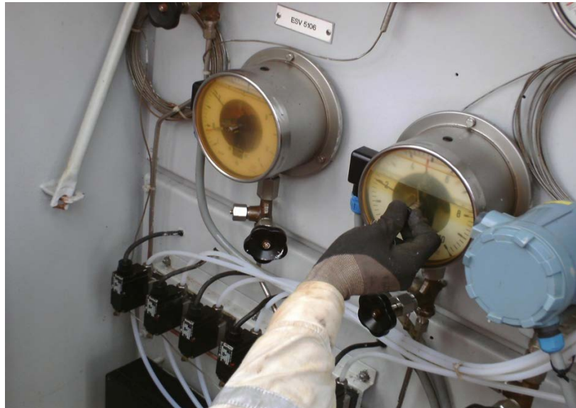
Figure 5-16 Testing of the high/low pressure alarm using a special handle
