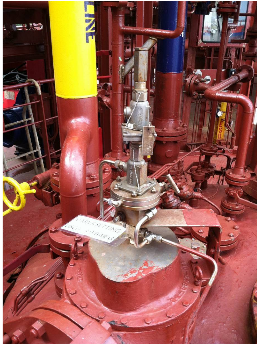
Figure 8-11 MARVS stacked correctly, typical LPG set-up
