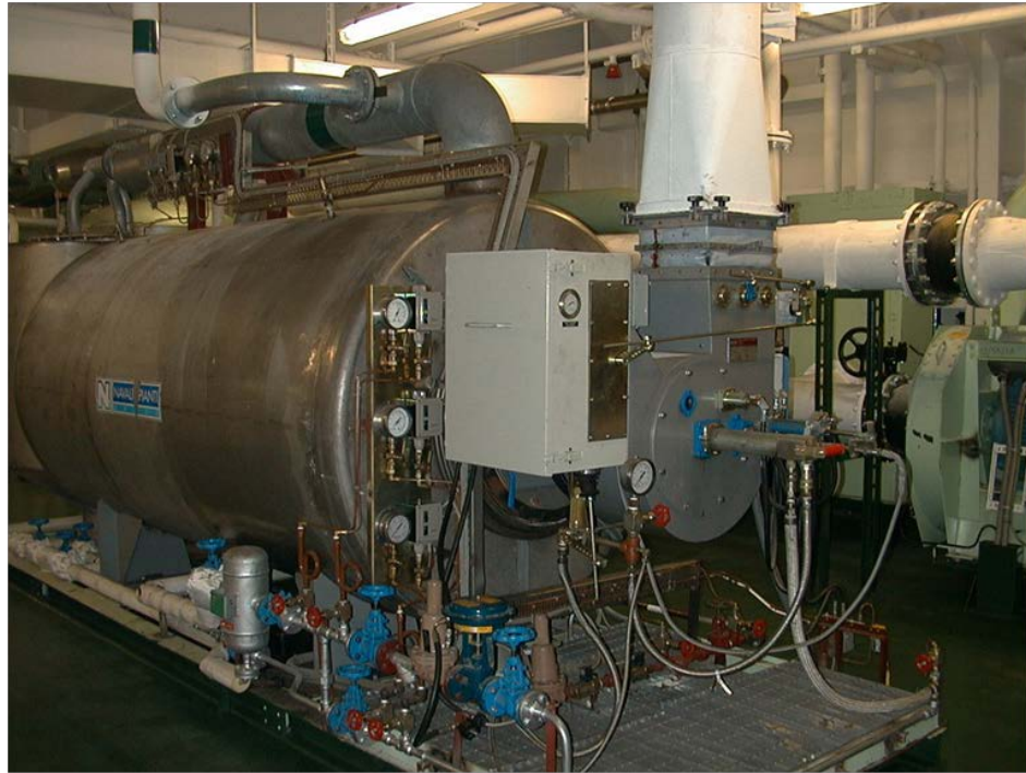
Figure 9-1 IGS on a gas carrier
