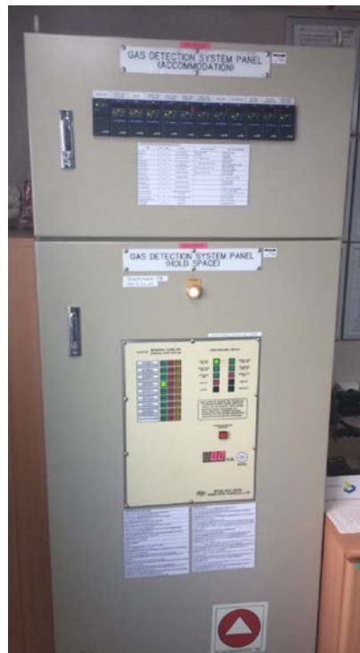
Figure 5-5 Combined suction (holds/un-manned spaces)/electronic (accommodations/manned spaces) fixed gas detection system
