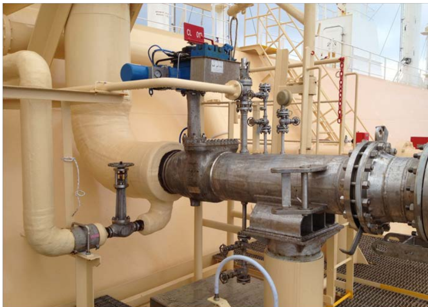
Figure 8-2 Typical ESD valve
