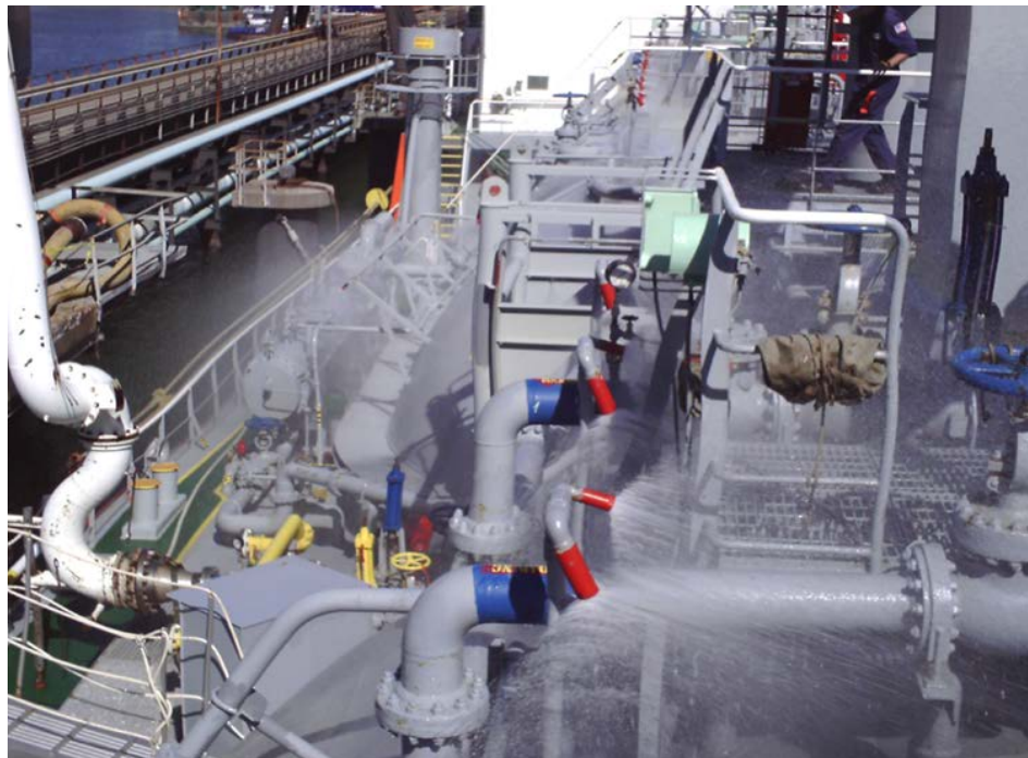
Figure 14-1 Activated deck water spray system (manifold)
