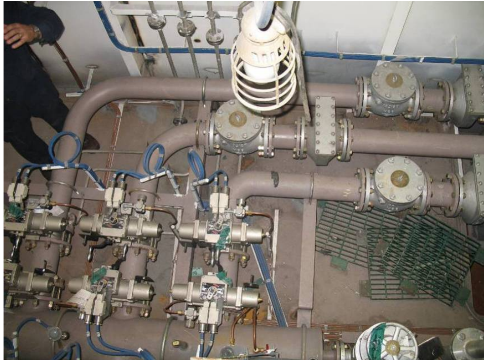
Figure 13-6 Multiple valve arrangements
