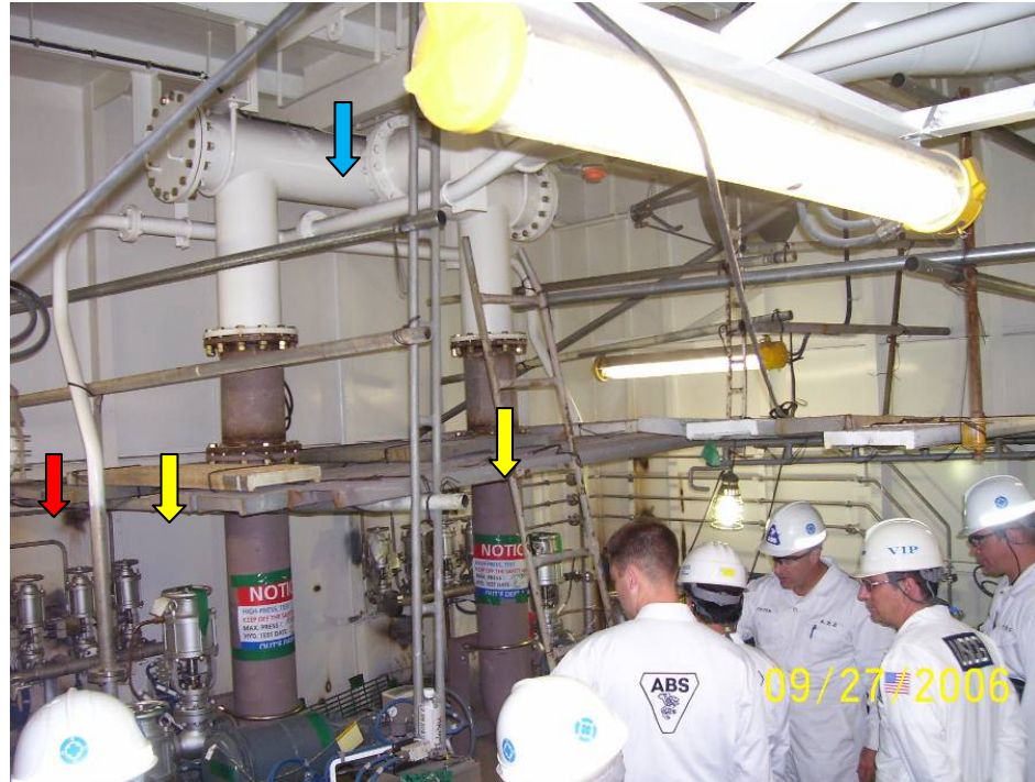
Figure 13-7 Fail-open vent valves
