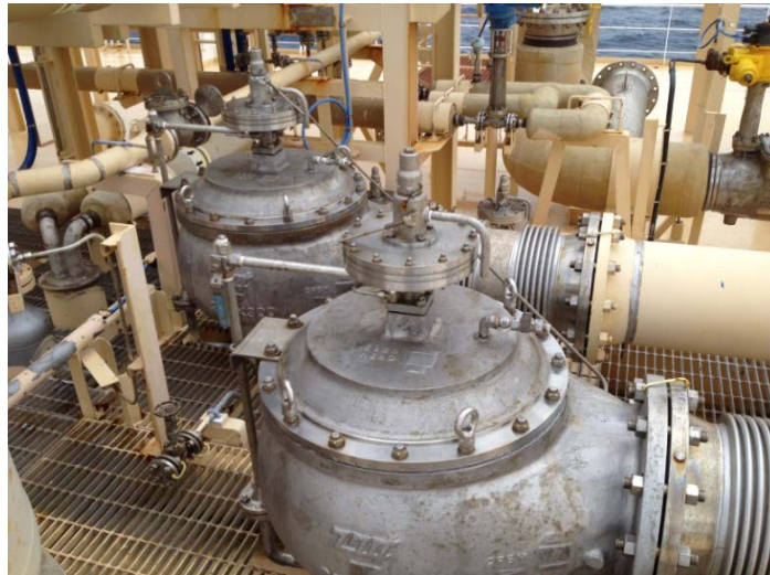
Figure 8-8 Cargo relief valves
