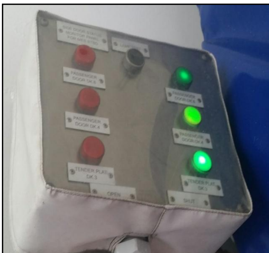
Shell Opening Indicator Panel at MES Station
