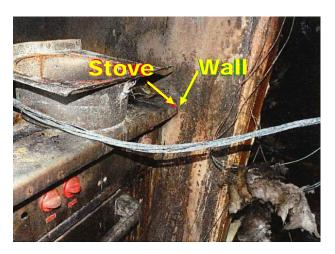
Per the appliance's rear data plate, the recommended safe clearance between the appliance and combustible construction material is six inches. The actual clearances to the adjacent walls, which were made of combustible wood and fiber-reinforced plastic, were one inch from the appliance's side and less than an inch from its rear. Moreover, the wall surfaces were covered with stainless steel sheet metal, which conducted the appliance's heat and caused the walls to ignite.
