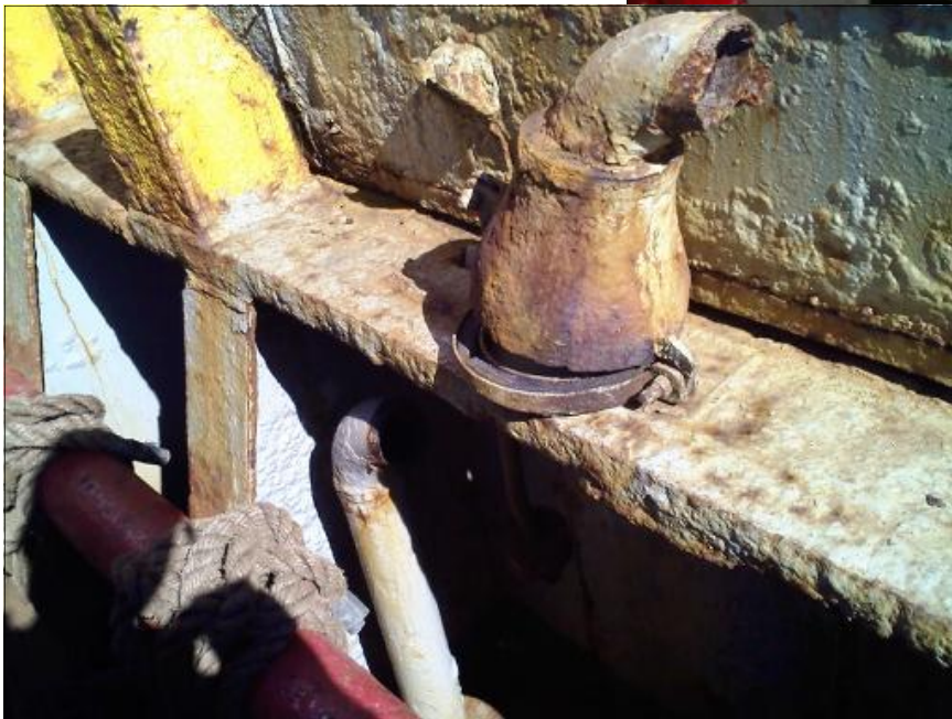
Top: Malfunctioning smoke detector, wrapped in plastic to prevent recurring alarm sounding (USCG Sector Honolulu) Right: Blocked fuel valve preventing remote actuation (USCG Sector New Orleans). Bottom: Significant corrosion and wastage on gooseneck vent.
