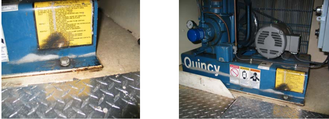
Figure 44. One company intends to reduce noise and vibration by replacing these current compressor mounts with sound-deadening ones.
